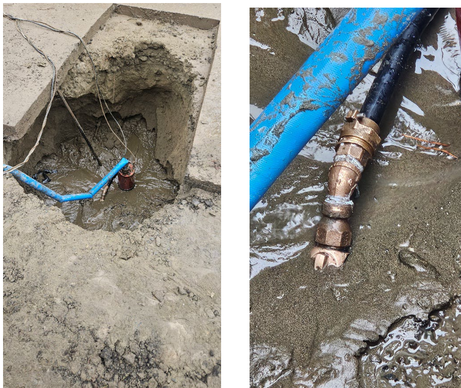
A ¾ poly service lateral ruptured on Holly Drive (before and after):
