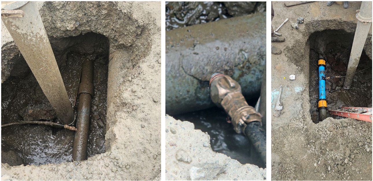
A ¾ poly service lateral ruptured on Holly Drive (before and after):
