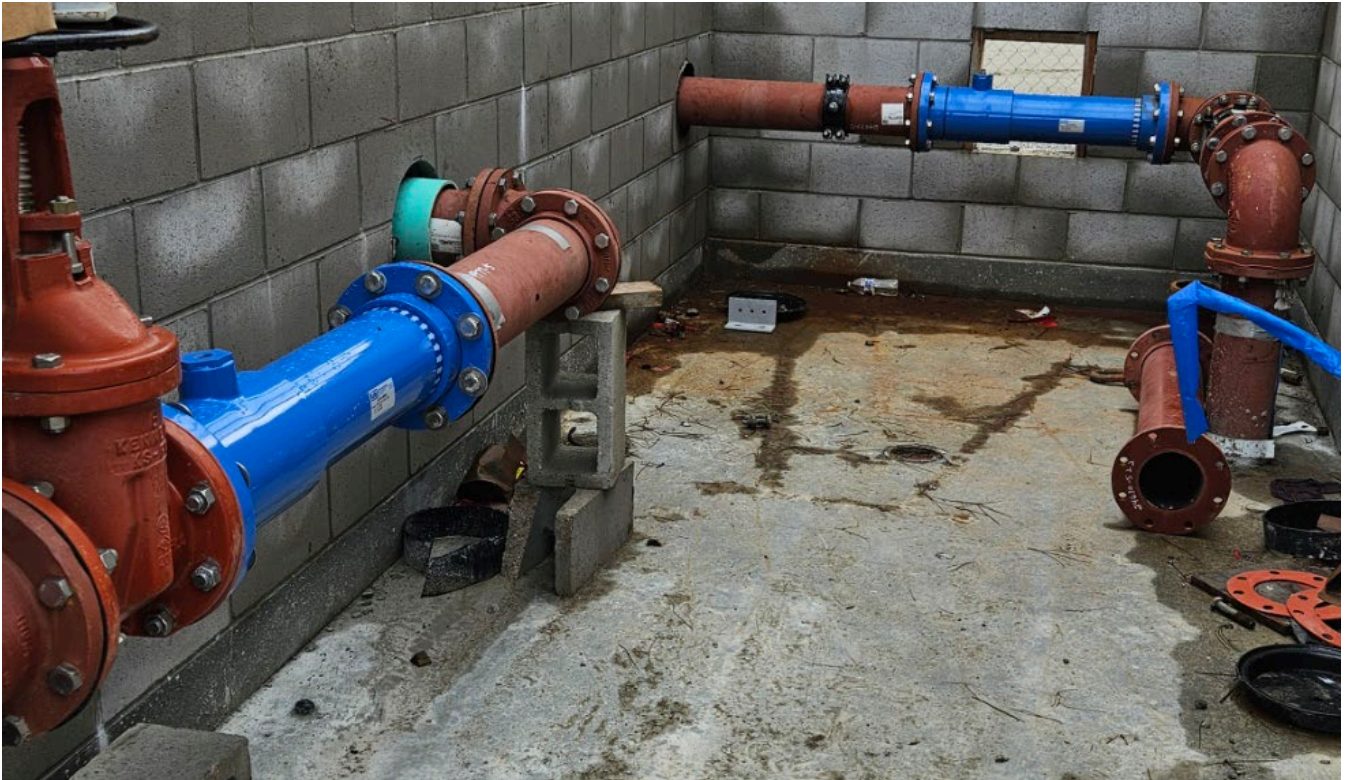
6" mixers in chlorinator room (in process)
