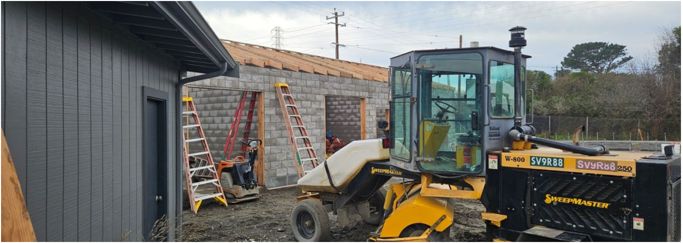
1901 Park Street Pumphouse as of January 7, 2025
