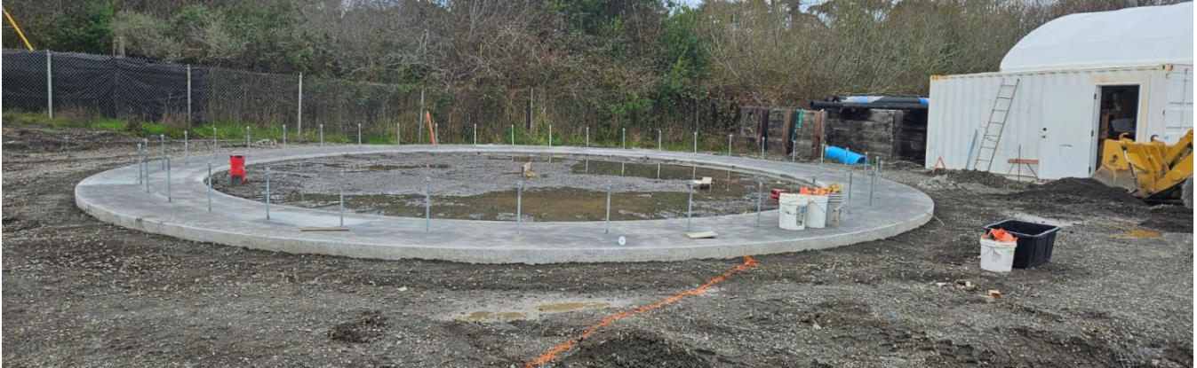
New Tank Foundation: Panels arriving Late January/February 2025
