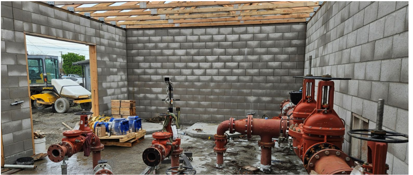
Interior of pumphouse with roof underway
