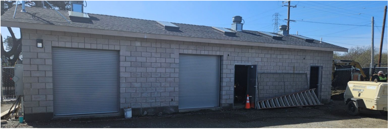
1901 Park Street Pumphouse as of March 11, 2025
