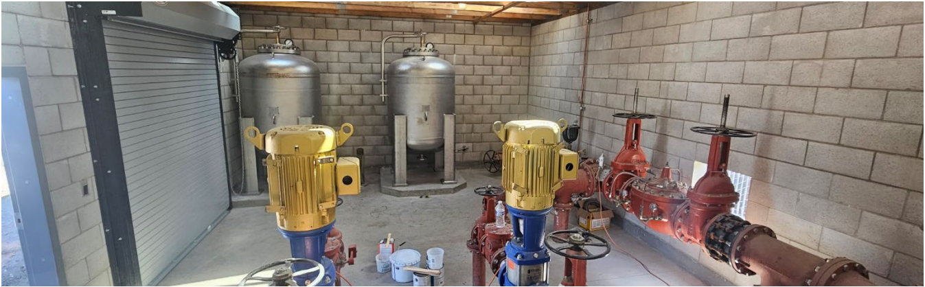
Inside pumphouse facing east
