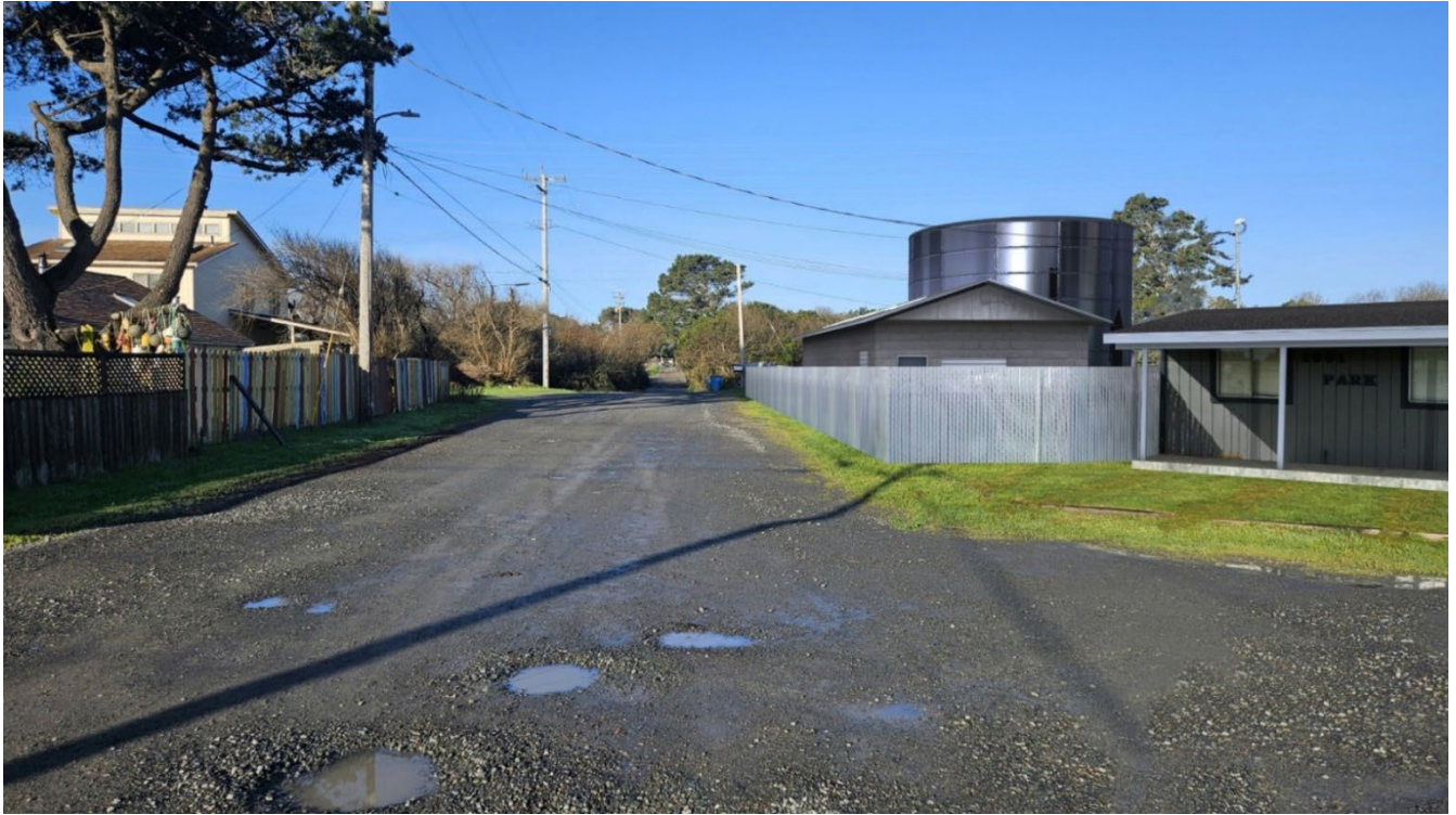
New Tank/Pump Station Simulation. Tank is 31' tall Gas Fused Bolted Steel
