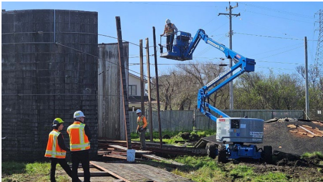
Redwood Storage Tank Staves Being Removed
